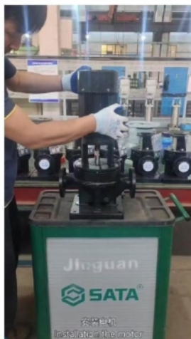
安装电机 Installation the motor.
