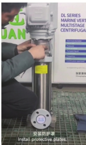
联轴器两侧缝隙一致 Ensure the clearance of coupling block is consistent
