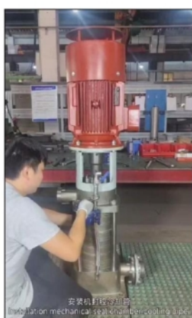
安装机封冷却管 Installation mechanical seal chamber cooling pipe.
