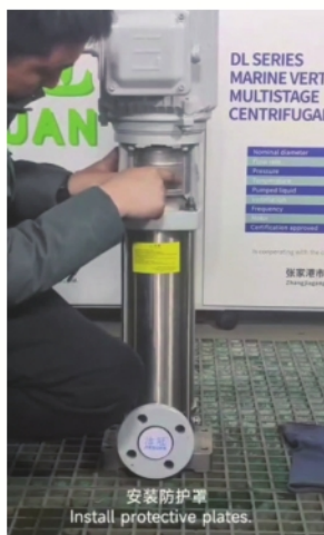
安装防护罩 Install protective plates.
