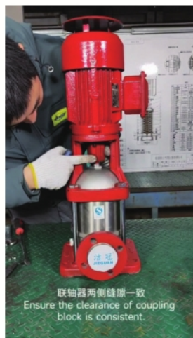
联轴器两侧缝隙一致 Ensure the clearance of coupling block is consistent.
