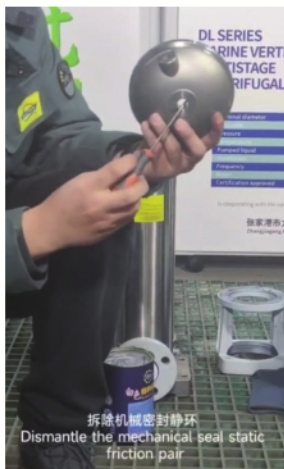
拆除机械密封静环 Dismantle the mechanical seal static friction
