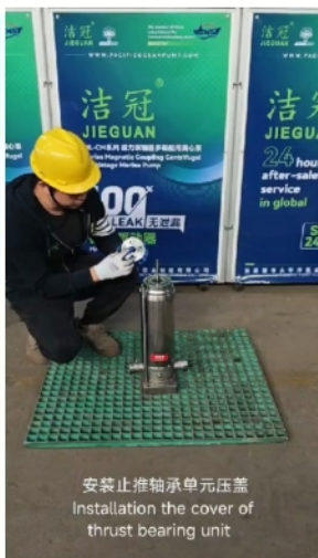
安装止推轴承单元压盖 Installation the cover of thrust bearing unit
