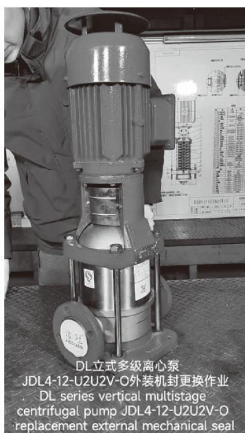
DL立式多级离心泵 JDL4-12-U2U2V-O外装机封更换作业 DL series vertical multistage centrifugal pump JDL4-12-U2U2V-O replacement external mechanical seal
