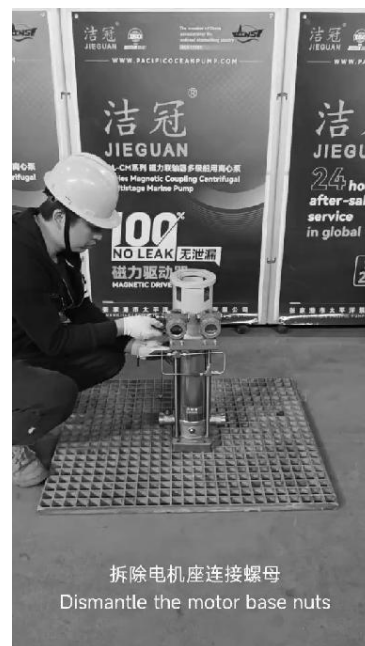
拆除电机座连接螺母 Dismantle the motor base nuts
