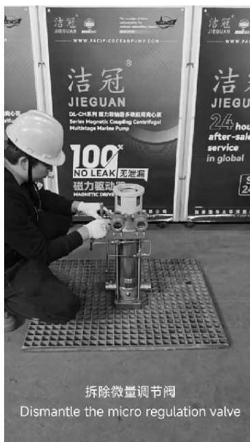
拆除微量调节阀 Dismantle the micro regulation valve
