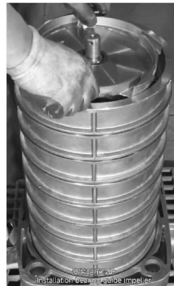
安装轴承导叶 Installation bearing guide impeller.
