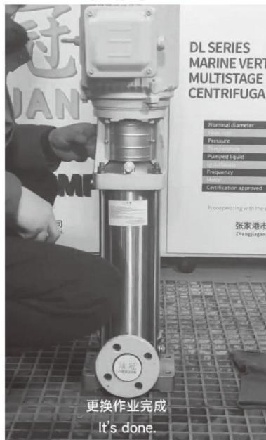
更换作业完成 It's done.
