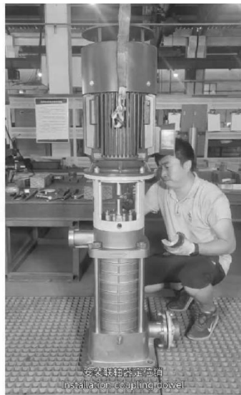
安装联轴器定位销 Installation coupling dowel.
