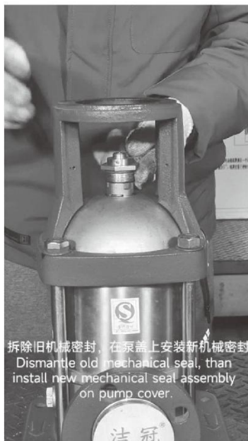
拆除旧机械密封，在泵盖上安装新机械密封 Dismantle old mechanical seal, then install new mechanical seal assembly on pump cover.
