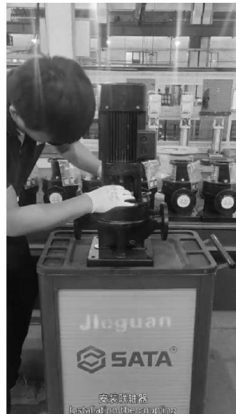
安装联轴器 Installation the coupling.
