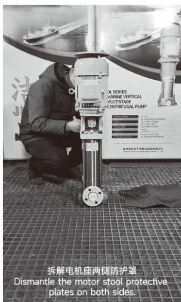
拆解电机座两侧防护罩 Dismantle the motor stool protective plates on both sides.
