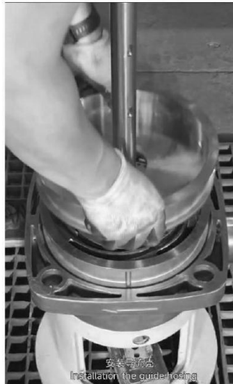
安装导流壳 Installation the guide housing.
