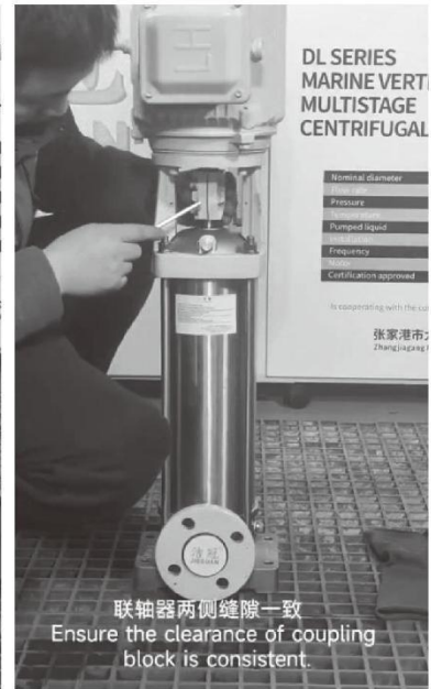
联轴器两侧缝隙一致 Ensure the clearance of coupling block is consistent.
