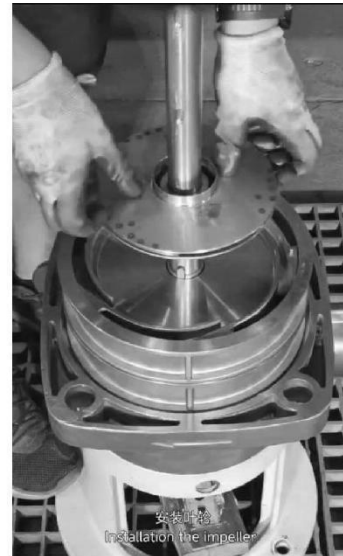
安装叶轮 Installation the impeller.
