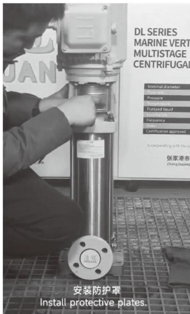
安装防护罩 Install protective plates.
