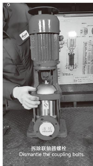
拆除联轴器螺栓 Dismantle the coupling bolts.
