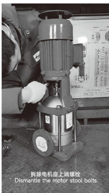
拆除电机座上端螺栓 Dismantle the motor stool bolts.
