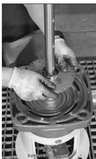
安装叶轮 Installation the impeller.
