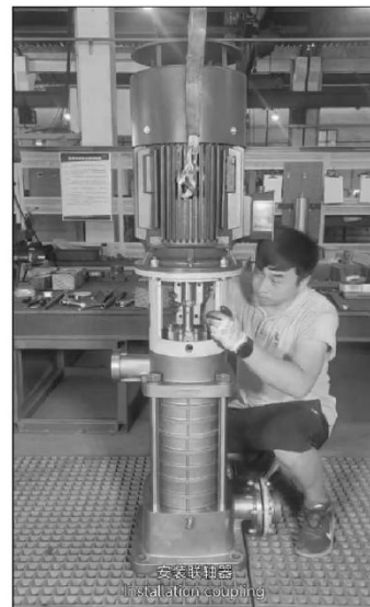
安装联轴器 Installation coupling.
