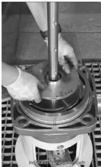
安装叶轮 Installation the impeller again.
