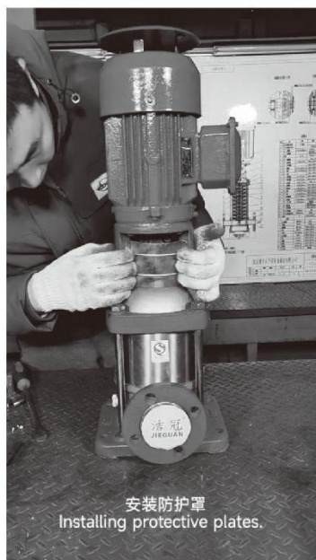
安装防护罩 Installing protective plates.
