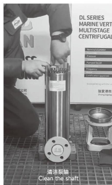
清洁泵轴 Clean the shaft
