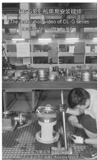
在泵轴上安装叶轮平键 Installation impeller key on the shaft.
