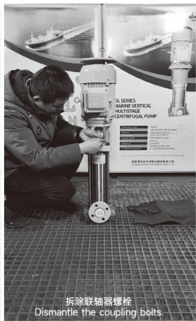
拆除联轴器螺栓 Dismantle the coupling bolts.
