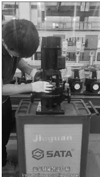
安装联轴器定位销 Installation coupling dowel.
