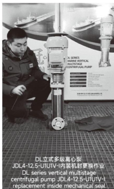
DL 立式多级离心泵 JDL4-12.5-U1U1V-I 内装机封更换作业 DL series vertical multistage centrifugal pump JDL4-12.5-U1U1V-I replacement inside mechanical seal
