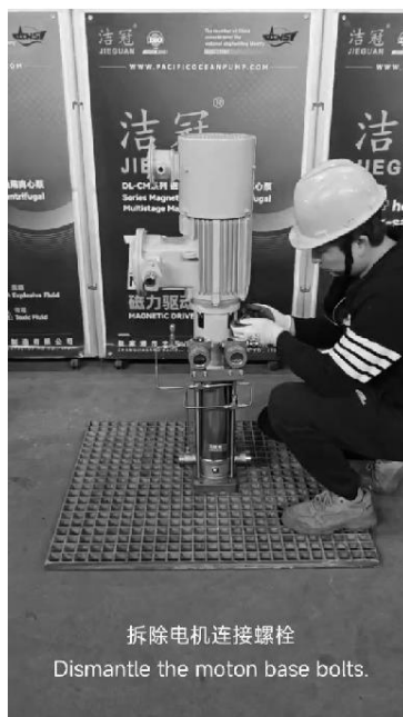
拆除电机连接螺栓 Dismantle the motor base bolts
