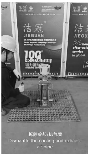
拆除冷却/排气管 Dismantle the cooling and exhaust air pipe
