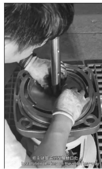
将平键安装到泵轴槽口处 Installation the key on the shaft key-way. Key-way.
