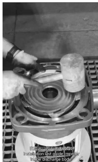
在泵出口段安装末级导叶 Installation last guide impeller in the discharge body.
