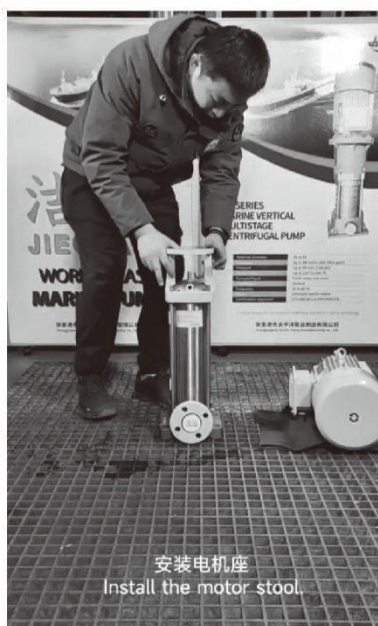
安装电机座 Install the motor stool.
